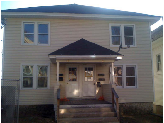
Mountain Avenue—Project Home
